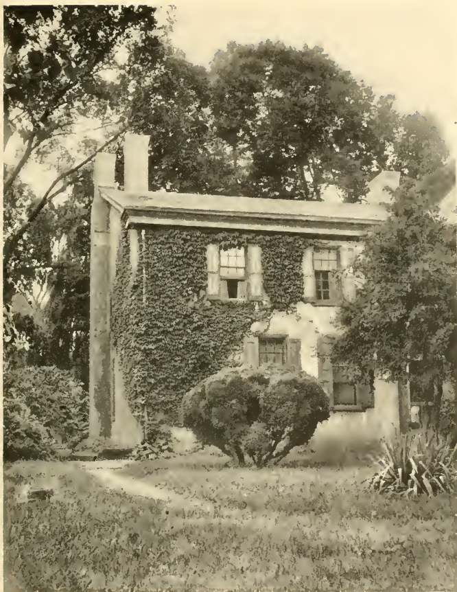
REAR VIEW OF RIDGELY HOUSE FROM THE GARDEN. (BUILT 1728.)
